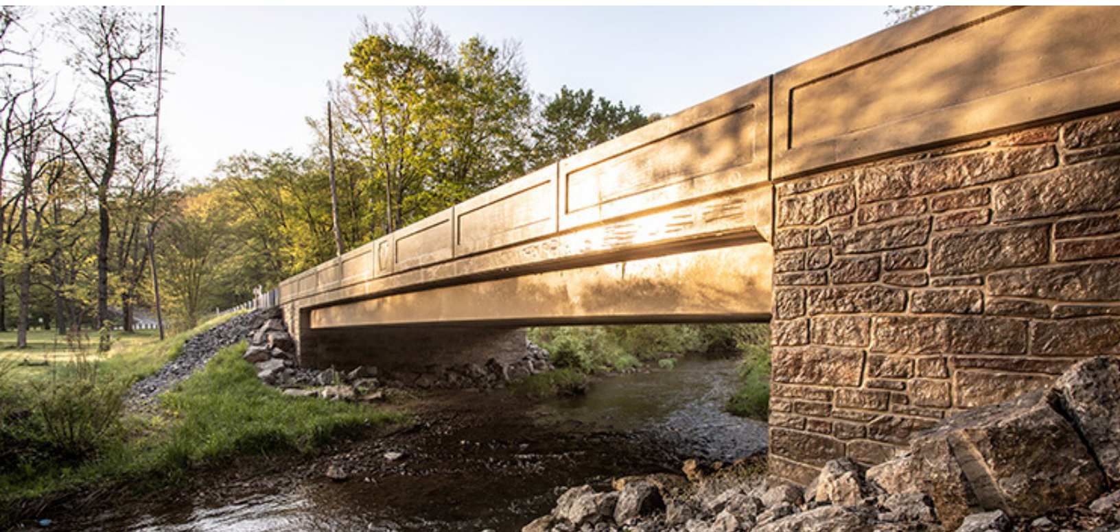
Bridges in the Pennsylvania Rapid Bridge Replacement Program incorporated innovative materials to protect their decks and extend their service, with structures designed for a 100-year lifespan.
