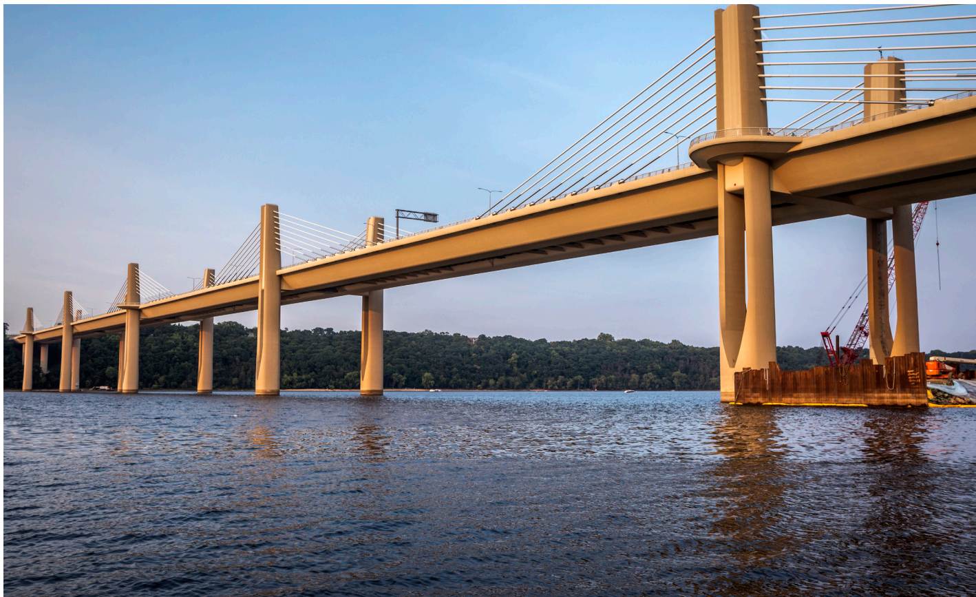
Collaboration on the St. Croix Crossing bridge led to a design that reduced the number of towers in the St. Croix River, a federally designated Wild and Scenic Riverway.
