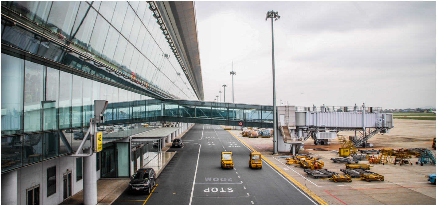
A holistic airport design takes airside operations into account in all other areas.
